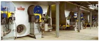
Example of a paper plant: 8 burners, 4 boilers, 2 fuels
