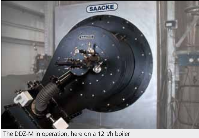
The DDZ-M in operation, here on a 12 t/h boiler
